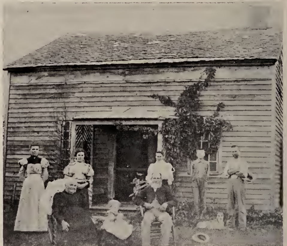
First weatherboard house built in Manchester Twp., Mich., by Benjamin R. Walworth, of sawed slabs and held together with wooden pegs.
