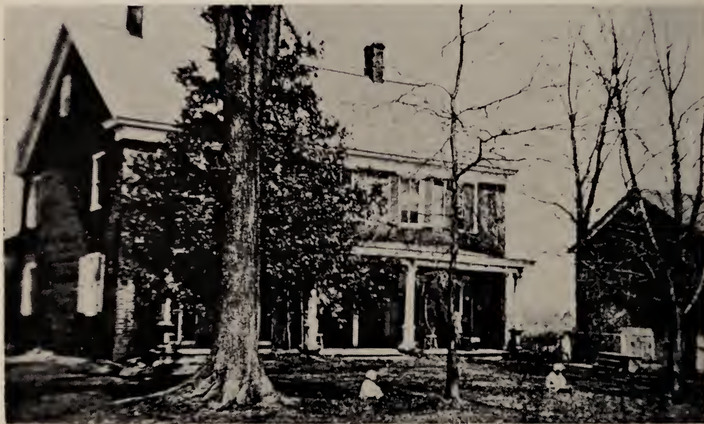
Built 1804 by Elisha Walsworth, Sr. #106 Photo. taken 1908.
